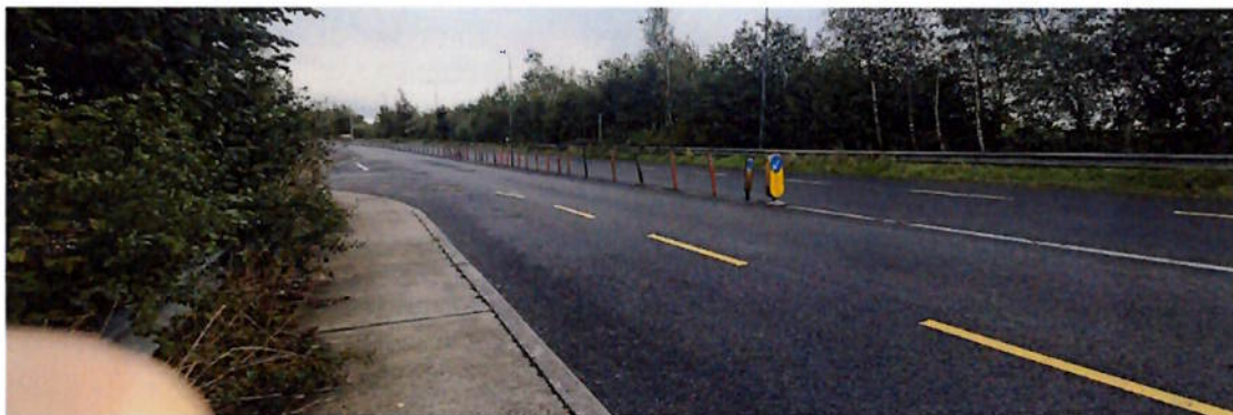
Wider view showing the length and continuity of the traffic-management measures.
