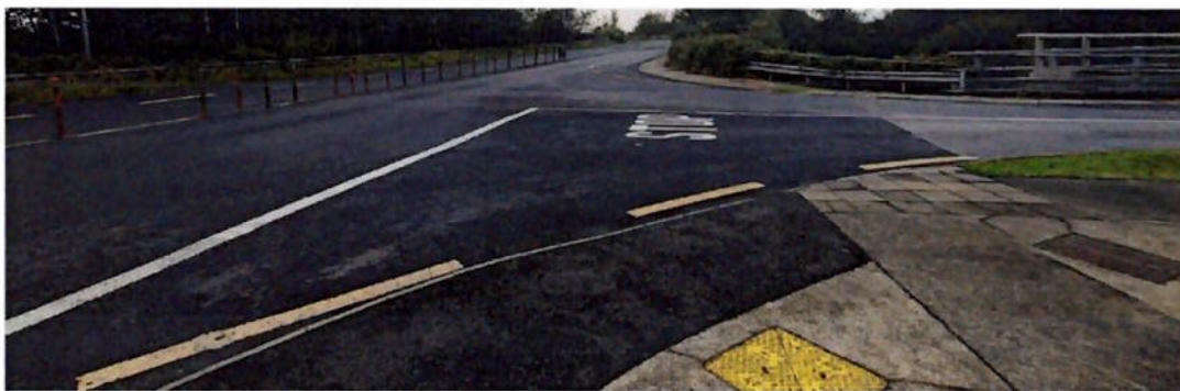
Wider context showing the surrounding road and access arrangement.
